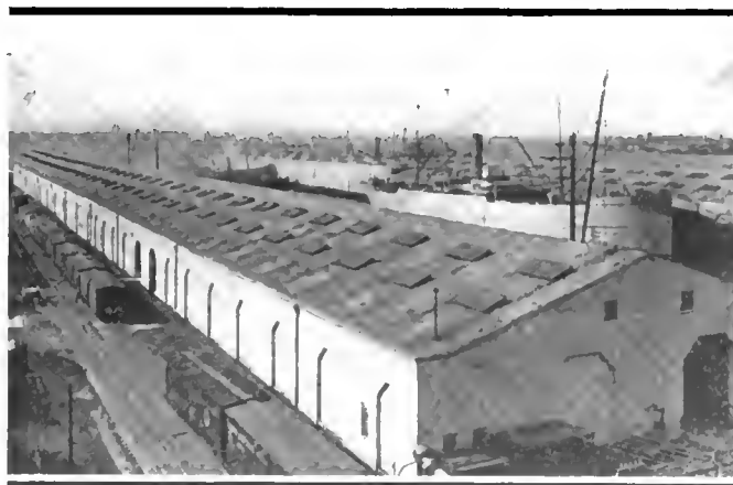
One of the covered docks at Bush Terminal. Ships on one side deliver the freight, cars on other side move it to its destination without the use of the city streets
